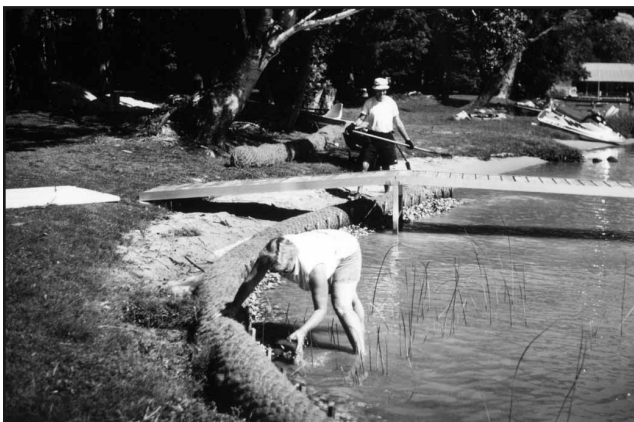
Figure 29: Hand adjustment of fieldstone along toe of coir.
