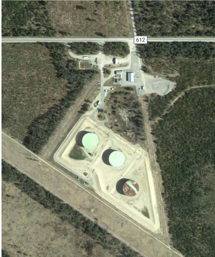
Figure 4-8: Lewiston Crude Oil Terminal
