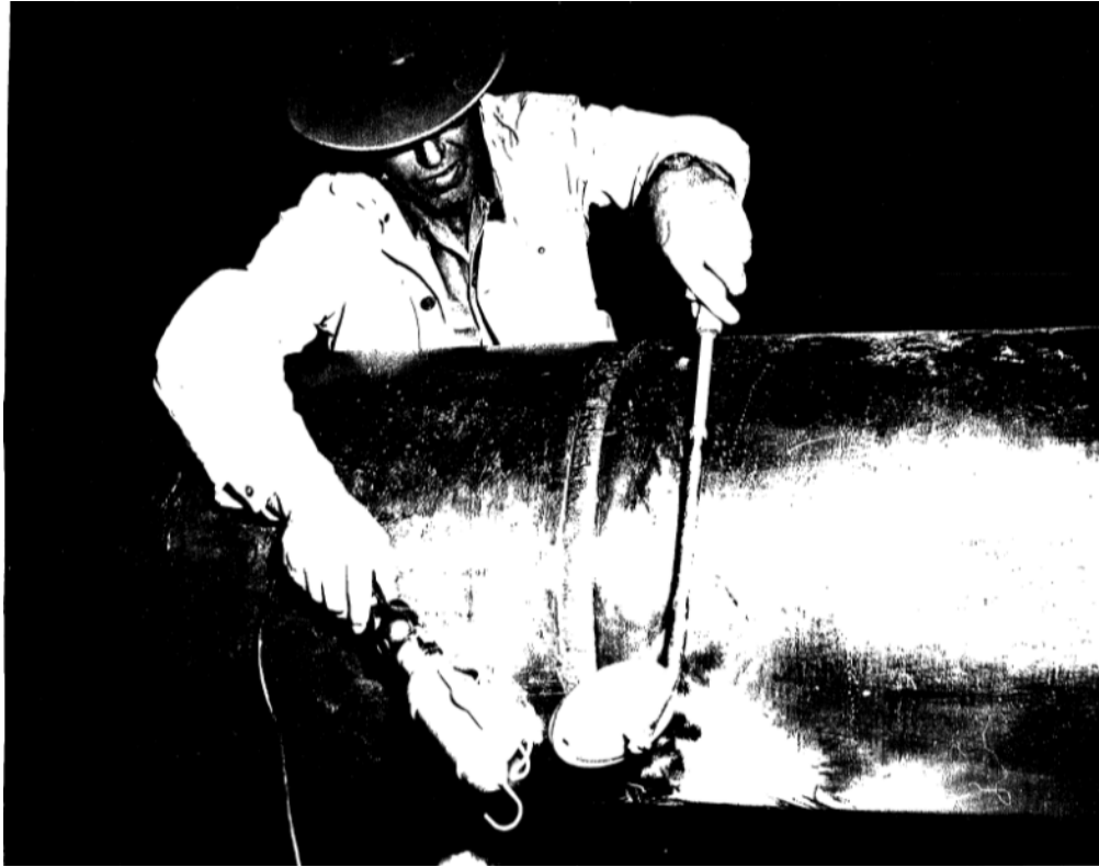
Figure 2-4: Visual Inspection of Girth Weld on Straits Pipe Segment
