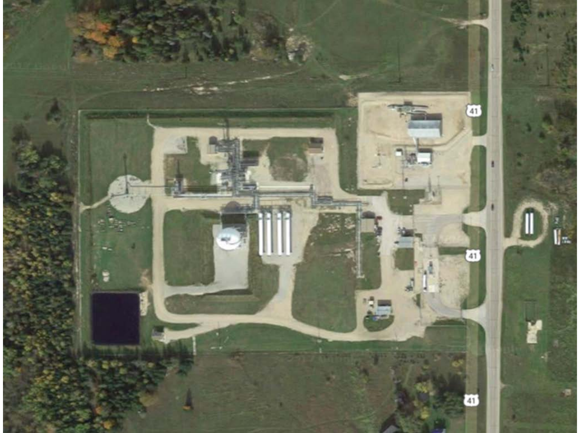
Figure 4-1: Rapid River Depropanizer Propane Distribution Terminal
