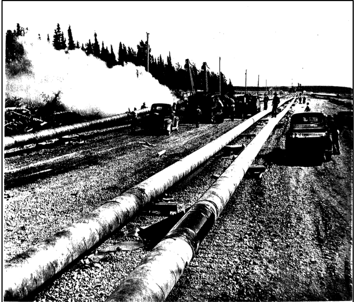
Figure 2-2: CTE-Coated Straits Crossing Segments
