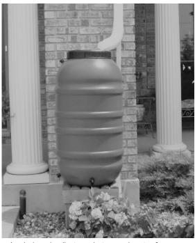
A rain barrel collects and stores rainwater from your rooftop which can be used for a variety of non-potable uses including watering your indoor plants and outdoor landscape. Using a rain barrel is a great first step to healthier rivers and streams in Northern Michigan.
