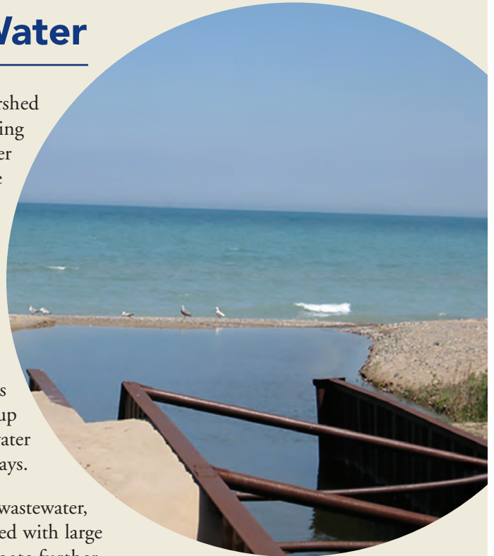
The Galbraith Drain takes water from the Forrest Manor subdivision near Port Huron to Lake Huron. The steel sheet piling is similar to the Butler Drain in Cheboygan.
