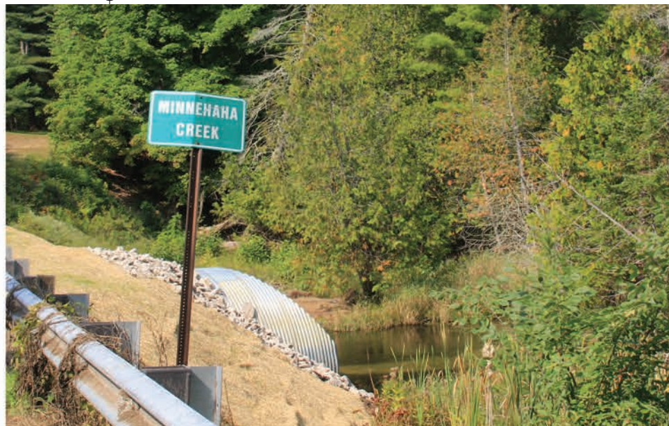
Geomorphology and habitat mapping were completed prior to removing and replacing the two undersized culverts that restricted flow and fish passage on Minnehaha Creek.
