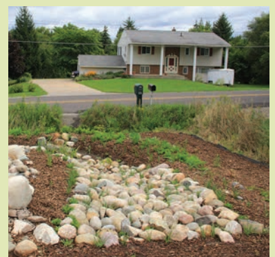
Rain gardens are specifically designed to address stormwater runoff on each property and vary in shape, size, and complexity.
