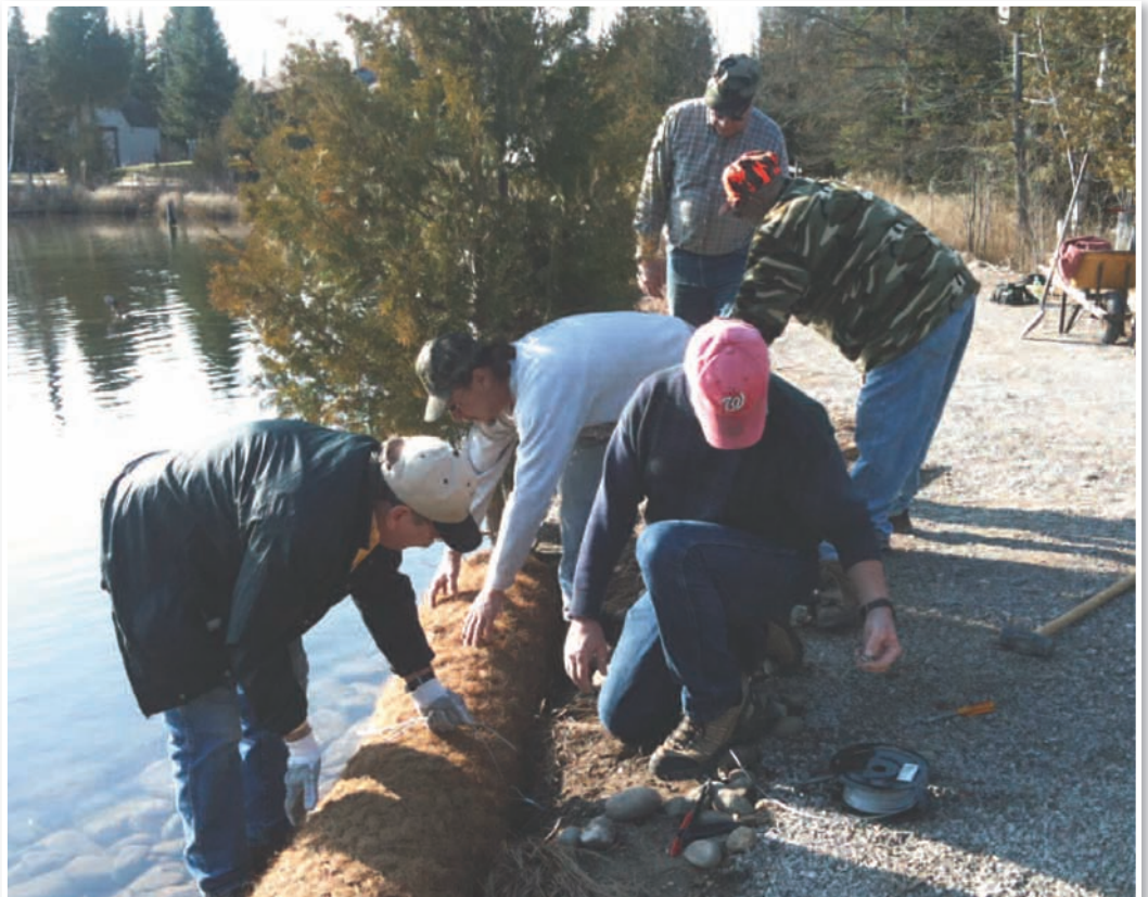
Twin Lakes Association volunteers work together to install a coir log at Owens Spillway. Their effort helped to stabilize and restore approximately 40 LF of shoreline.
