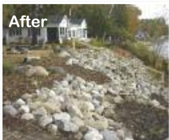
Native planting pockets are incorporated into fieldstone revetment.
