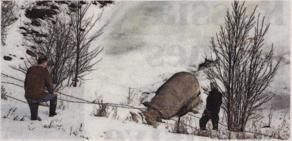
Part of the large earthen dam in the area of the Cheboygan Golf Course has eroded away, revealing a culvert, which is also in need of repair as a part of the Little Black River Watershed. PROVIDED PHOTO BY RON WILLIAMS
